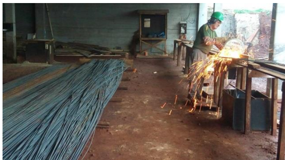
Figura 1. Cortando as ferragens.
