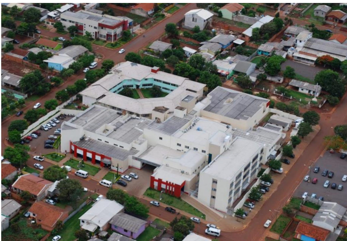
Figura 19: Vista Superior Hospital UOPECCAN.
