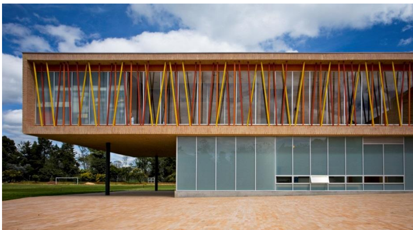
Figura 9: Fachada com brise-soleils.
