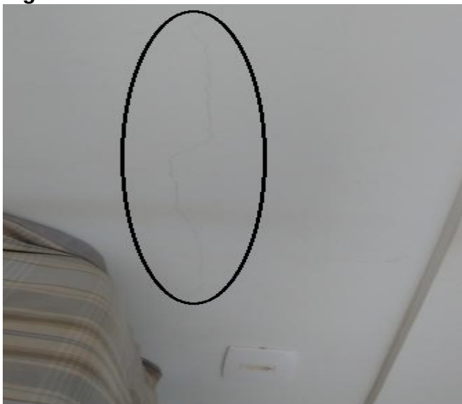
Figura 22 – Fissura vertical
