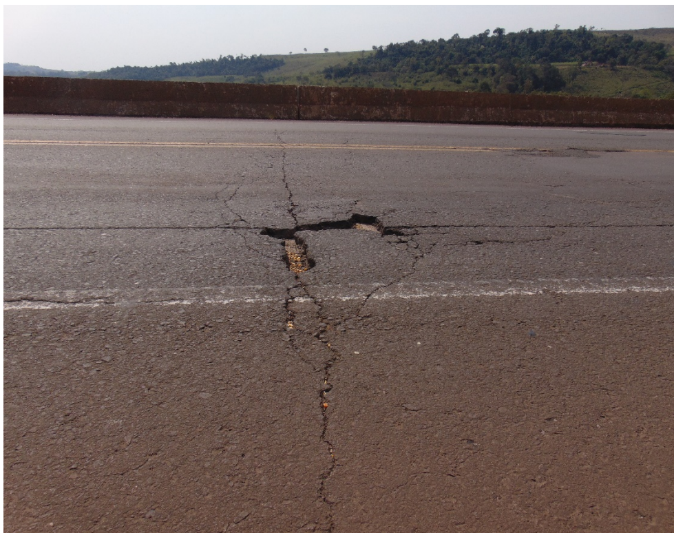
Figura 22: Painéis na laje principal
