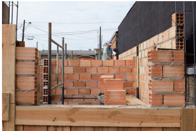
Figura 7 – Contraverga concretada
