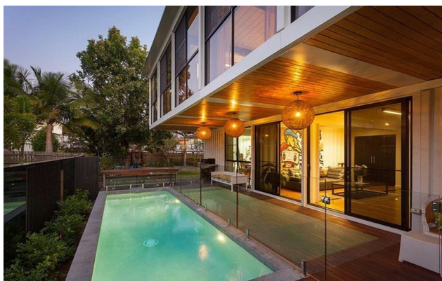
Figura 26: Uso de vidro 31 Shipping Containers Residence
