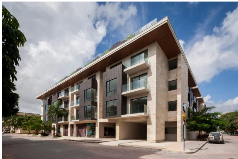
Figura 11: Fachada Hotel Boutique Cacao
