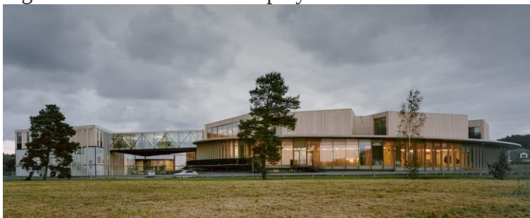
Figura 07. Vista fachada Exupery School
