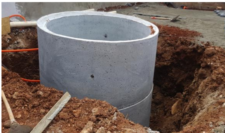
Figura 6: Cisterna executada in loco .
