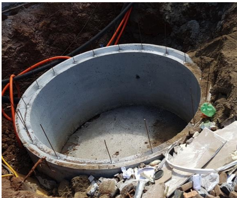
Figura 6: Cisterna executada in loco .
