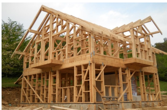
Figura 9 - Wood Framing
