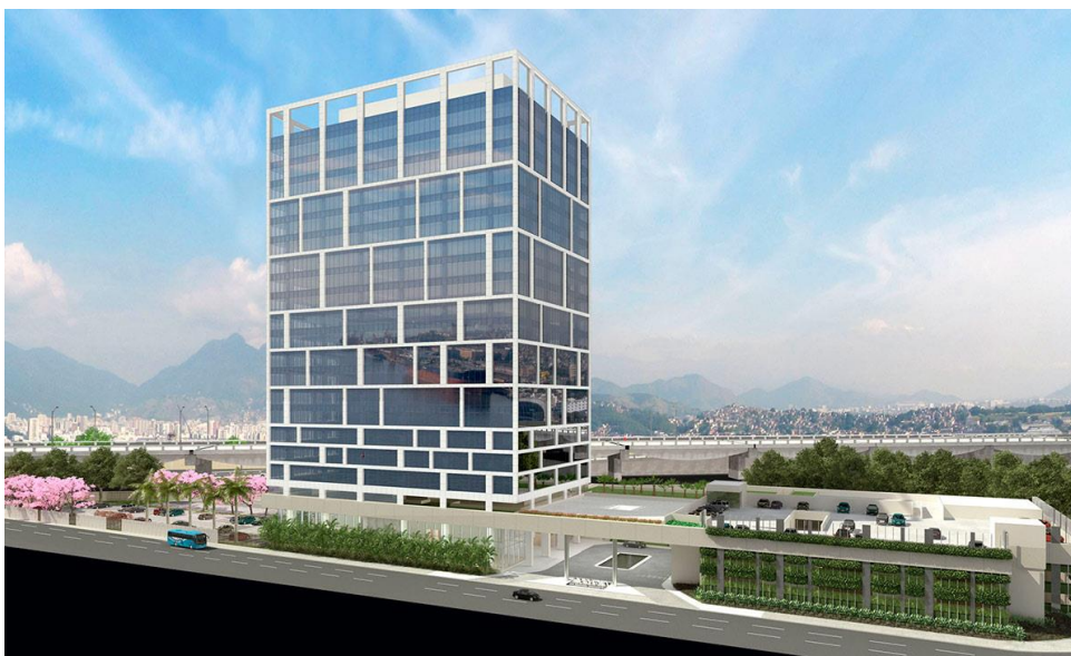
Figura 02: Port Corporate Tower
