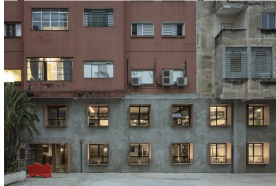
Figura 06 - Fachada Coworking Impact HUB
