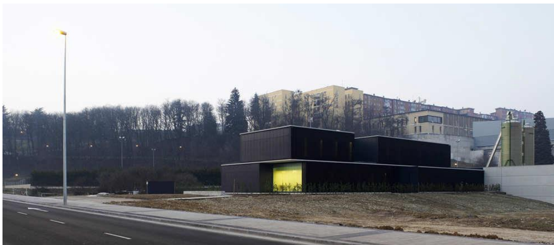
FIGURA06: Fachada do Shelter Home.
