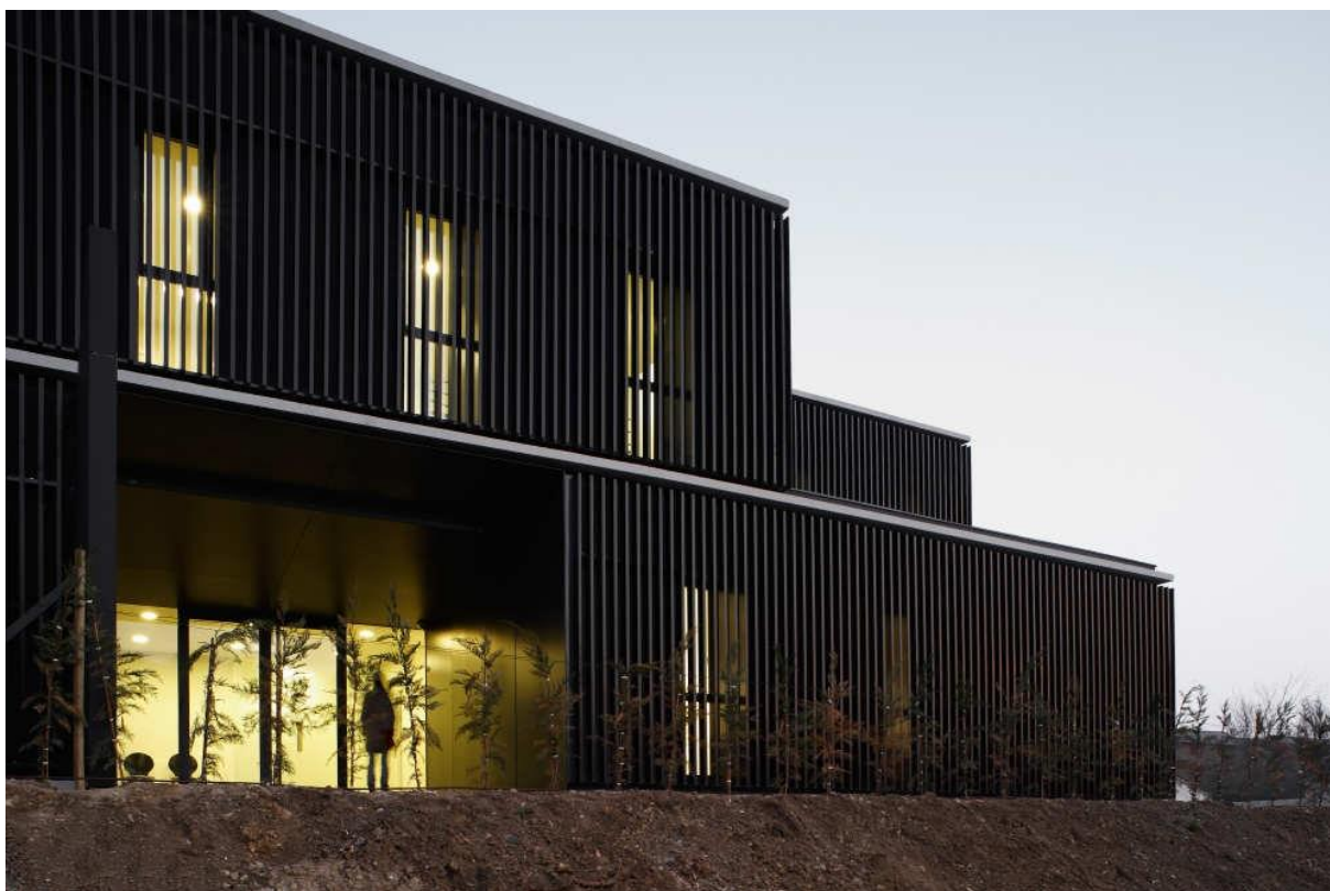
FIGURA 08: Fachada do Shelter Home.
