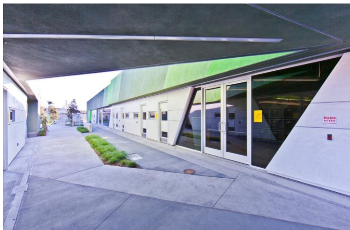
Figura 14: Exterior South Angels Care Center
