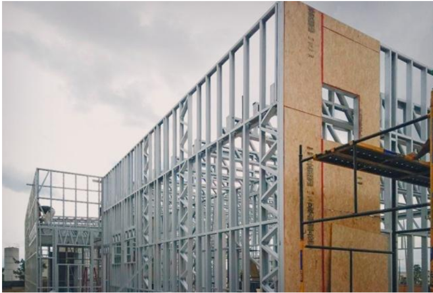
Figura 3: Steel framing
