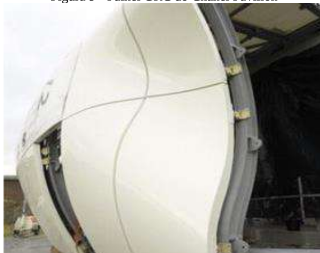
Figura 9 - Paineis GRC do Chanel Pavilion
