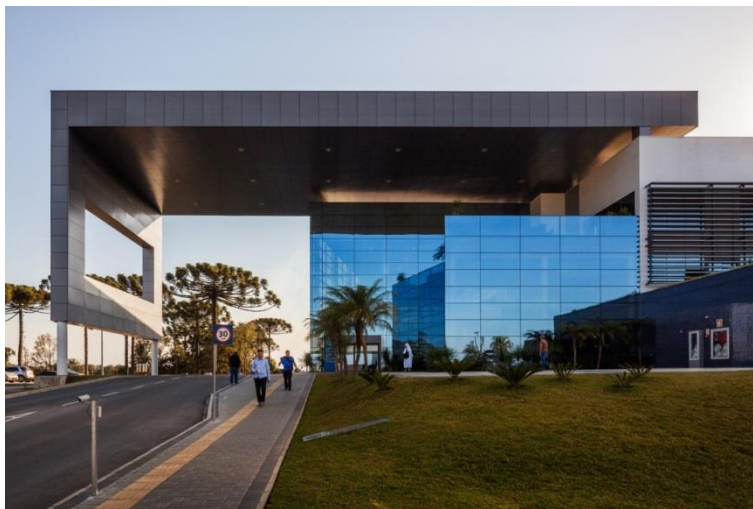
Figura 1 – Fachada principal Hospital do Rocio
