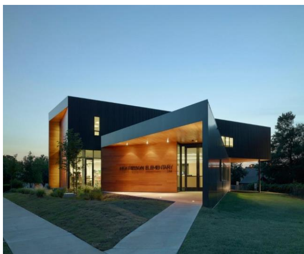
Figura 5 – Fachada – Montessori Elementary
