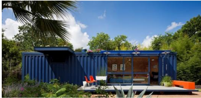
Figura 9: Volume Container Guest House
