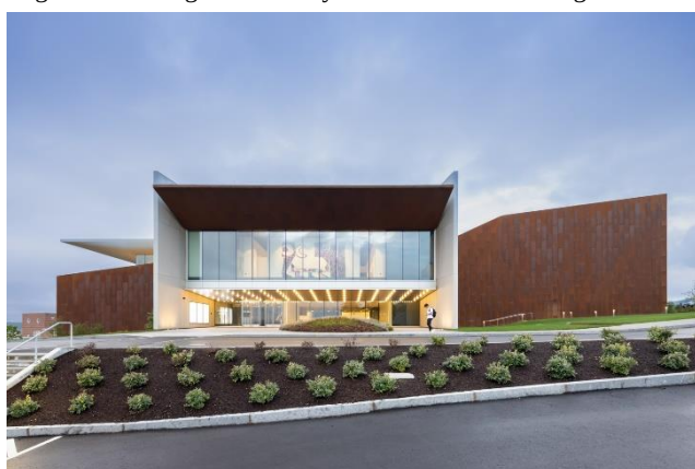
Figura 12: College of the Holy Cross Prior Performing Arts Center
