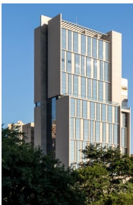
Figura 12 - Fachada - Wyndham Garden
