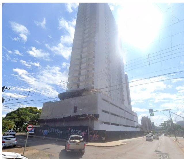
Embasamento Soleil Residence.
