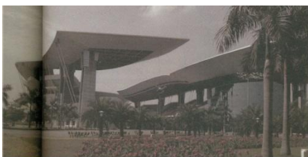
Fig.8. The Guangdong Olympic sports Center
